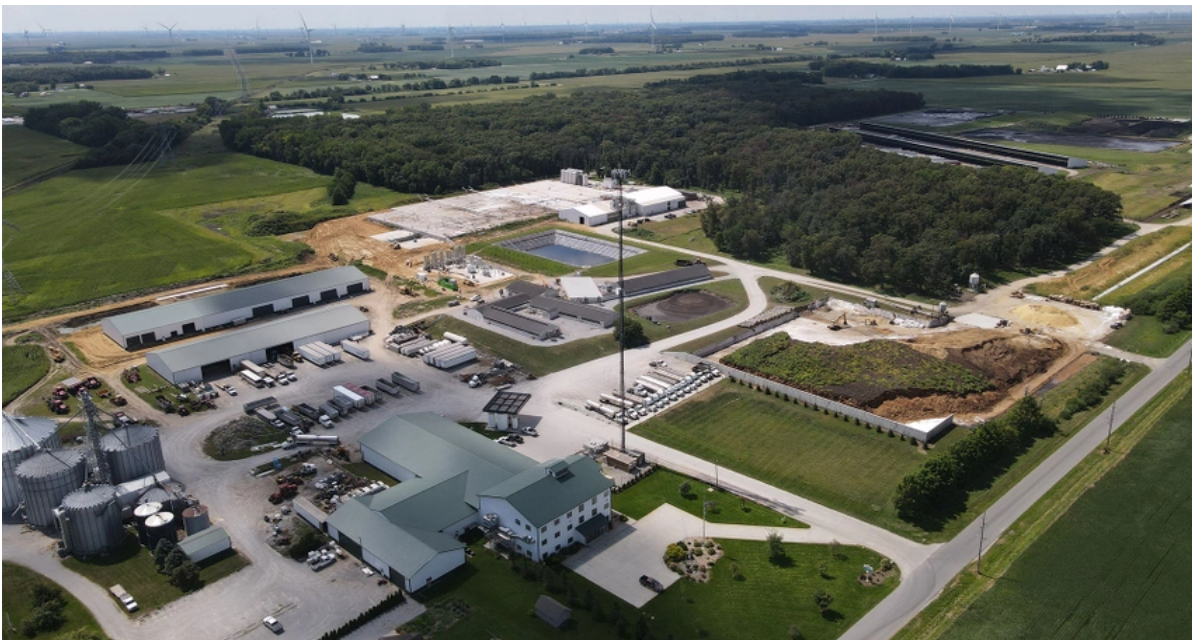
PRODUCING ENERGY: BioTown Ag, Reynolds, Ind., joined with Green Rock Energy Partners to form BioTown Biogas. This entity produces renewable energy — both electricity and renewable natural gas. BIOTOWN AG
