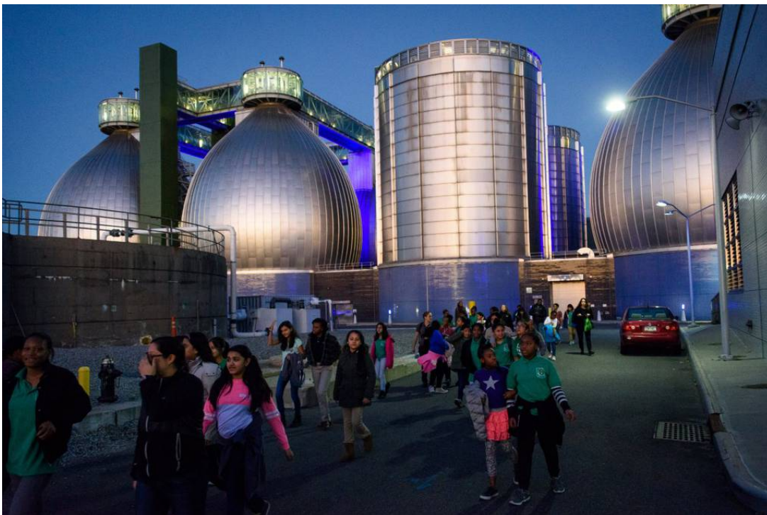
Newtown Creek Wastewater Treatment Plant in Brooklyn. (Gardiner Anderson/for New York Daily News)
