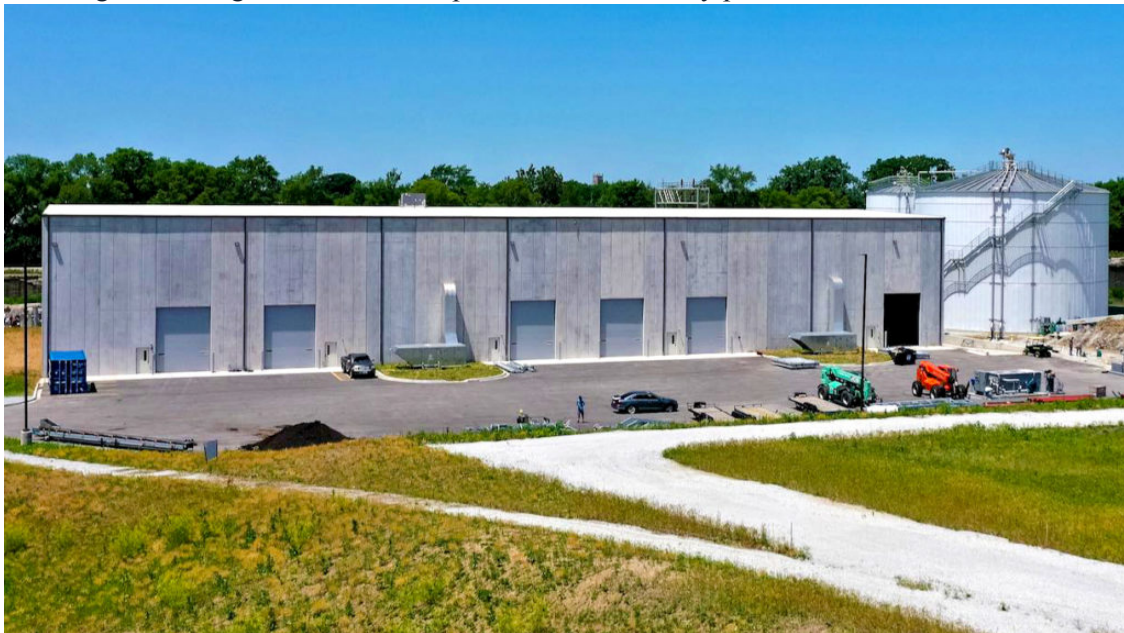
The Green Era AD and composting facility on Chicago's south side is built on a former brownfield site.
