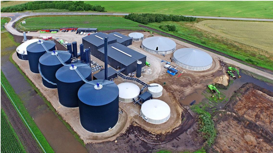
*Nature Energy anaerobic digestion facility produces RNG from livestock manure and source separated organics.*
