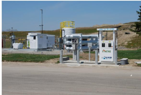
**In Michigan, landfill gas is being captured and upgraded into renewable compressed natural gas (R-CNG) to power vehicle fleets in the City of Riverview.**
