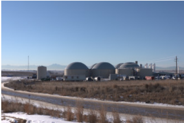
The Heartland Biogas facility in Weld County, Colorado. Rebecca Jacobson
