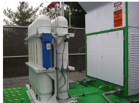
CNG storage bottles at the refueling station built and operated by Clean Energy for Central Jersey Waste’s refuse trucks
