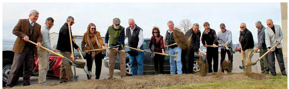
Public and private sector officials from Grand Junction and Mesa County Colorado break ground on the BioCNG gas refining system adjacent to the Persigo Wastewater Facility
