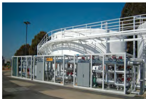
CleanWorld's Sacramento Bio-Digester is designed to process 100 tons of food waste per day
