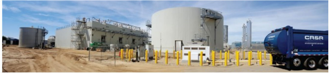
Phase 1 construction of CR&R's Food Waste-to-Vehicle Fuel Project
